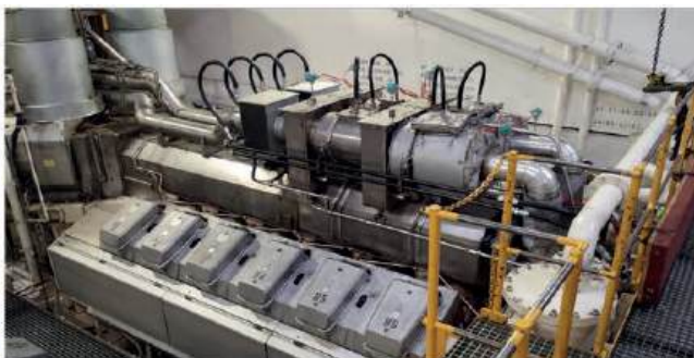
MS ARTANIA Wärtsilä 12V W32E engine - before and after E.G.R. installation
